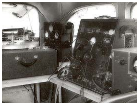
Disc-cutting equipment installed inside an automobile, used in Archive of Folk Song recording trips in the 1930s and 1940s. (American Folklife Center, Washington DC)
